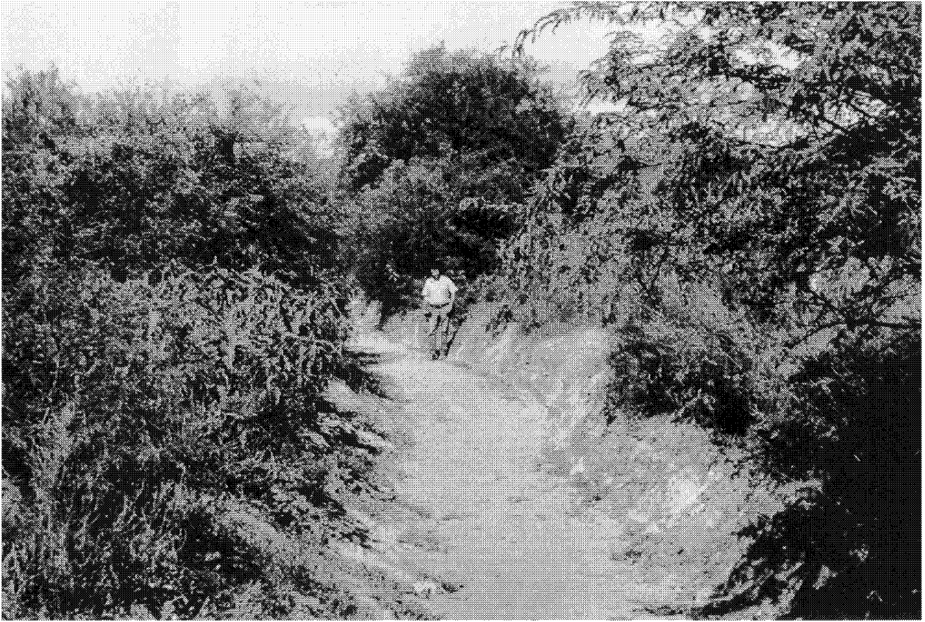
Figure 4.6. Canal carrying diverted floodwaters to multiple fields along a tributary of the Rio Sonora near Baviacora, Sonora.
