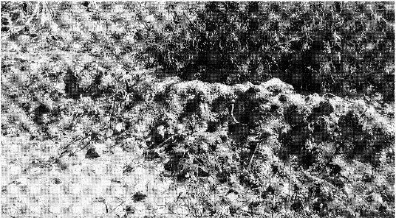
Figure 4.5. Earthen embankment for intrafield distribution of water along a tributary of the Rio Sonora near Baviacora, Sonora.
